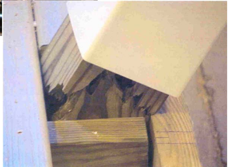
Photo 3: Post failure in bending just above joist.
